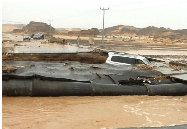
Figure 1. Failure of hydrological structur along the highway
