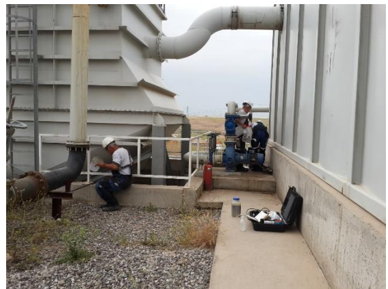
Figure3. The treated wastewater
